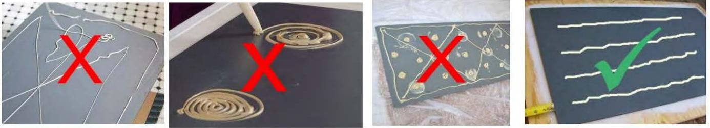
Mount mirror within 10 minutes of applying adhesive. Support mirror mechanically (mirror clips, etc.) until adhesive dries. Do not apply adhesive if the area temperature is below 15.5°C (60° F). Read and follow the AC035 adhesive instructions carefully.
